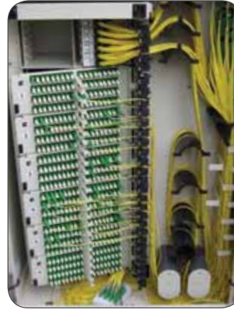
Correct Cable Routing
