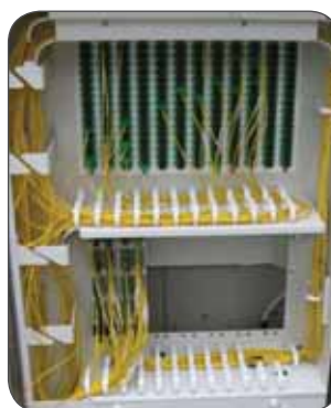
Figure 1. Poor Fiber Routing
