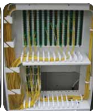
Figure 2. Correct Fiber Routing
