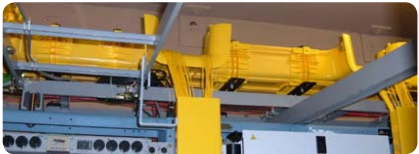
FiberGuide® Raceway securely routes and protects EATEL's valuable fibers
